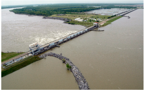
Low sill and Overbank Structures
