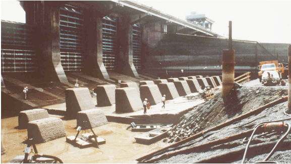
Outflow side view of the dewatered Low Sill under routine repair, 1987.
