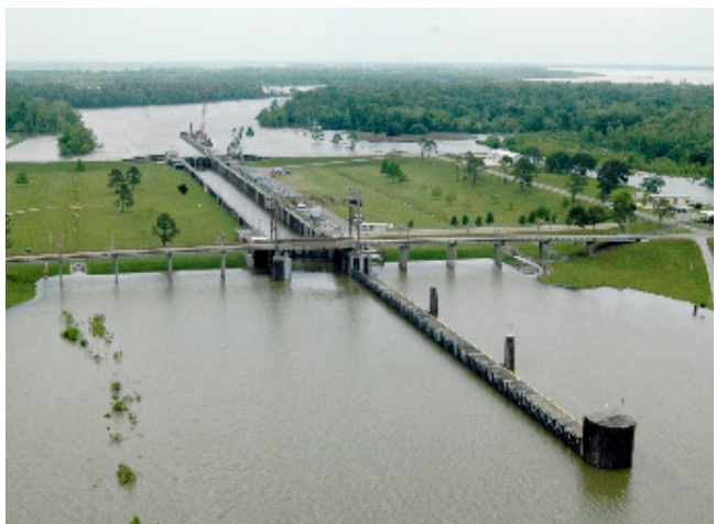
Old River Lock Structure
